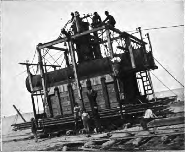
(a) Caisson on Rolls Ready to Launch.
